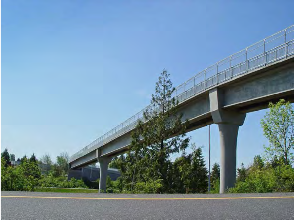
Prestressed Precast Concrete Girders
