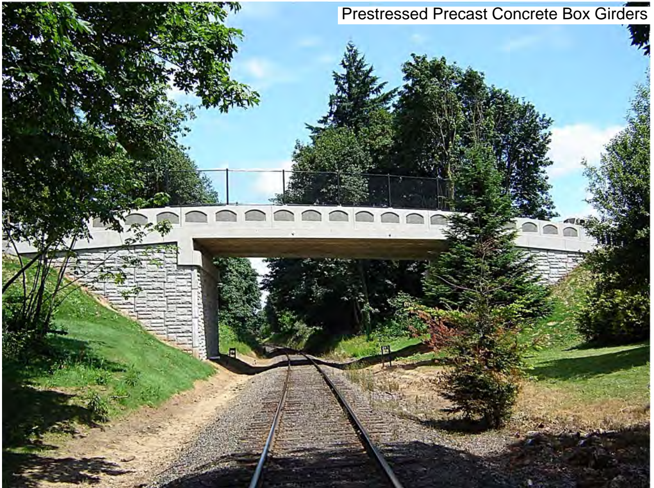
Prestressed Precast Concrete Girders
