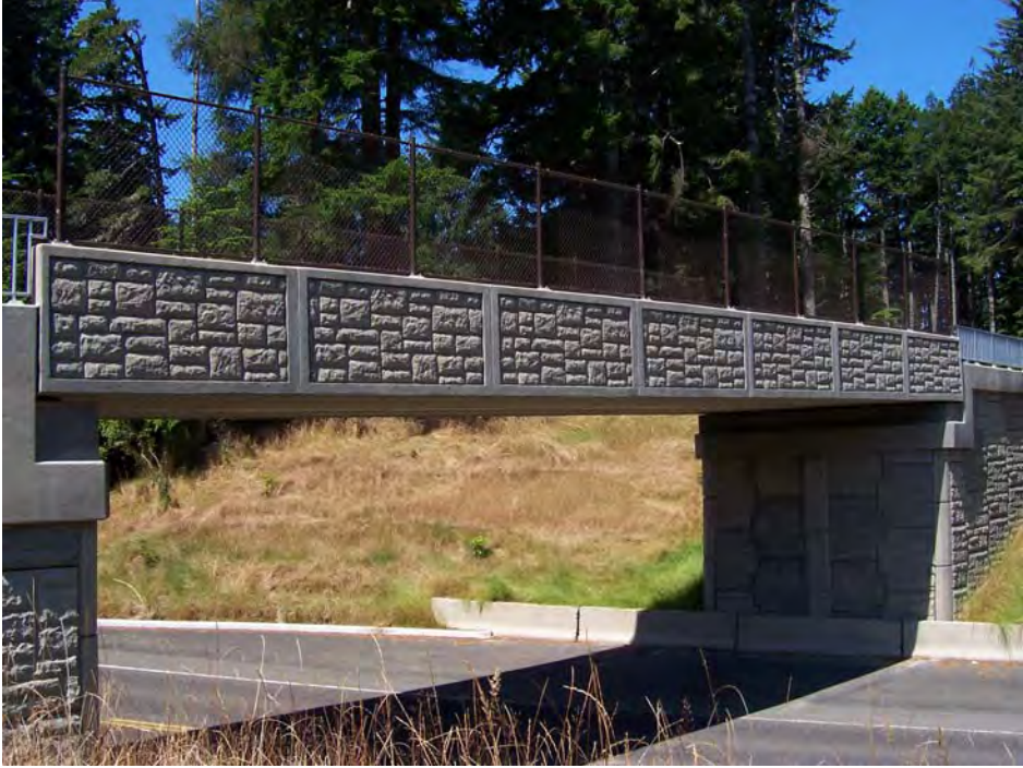
Prestressed Precast Concrete Box Girders
