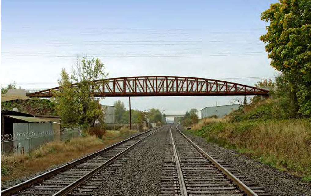
Steel Through Truss
